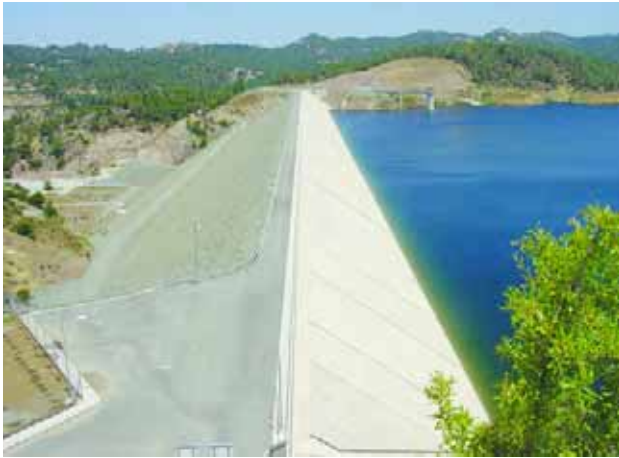
Kannaviou dam in operation
